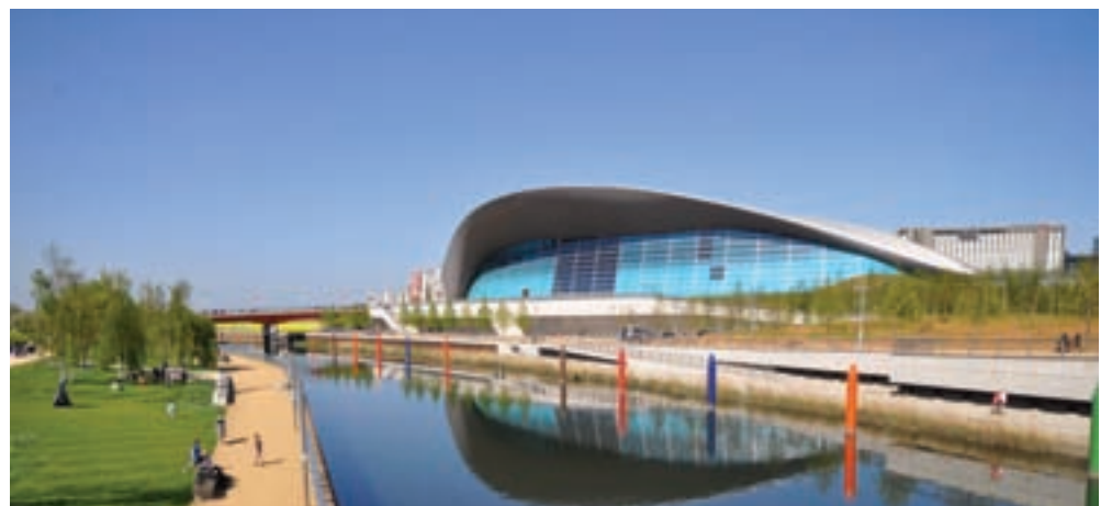
Aquatics Centre of the Queen Elizabeth Olympic Park in Stratford, East London
